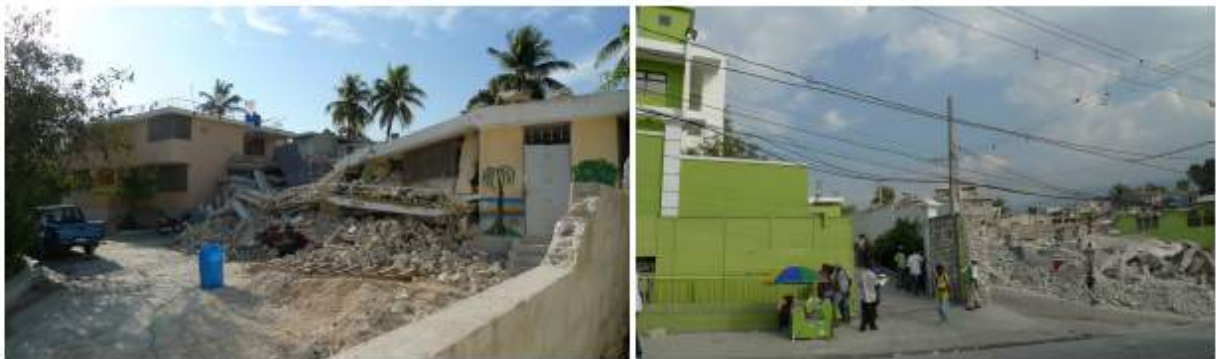
Figure 1a (left). Collapsed private school in central Port-au-Prince metropolitan region; a neighboring single-family house sustained no damage; (b, right) Well-built commercial building (left side) adjacent to catastrophic collapse of neighboring structure.
